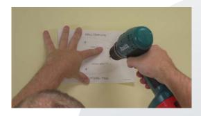
Remove the lid and fit the holder securely to the wall using three screws.
