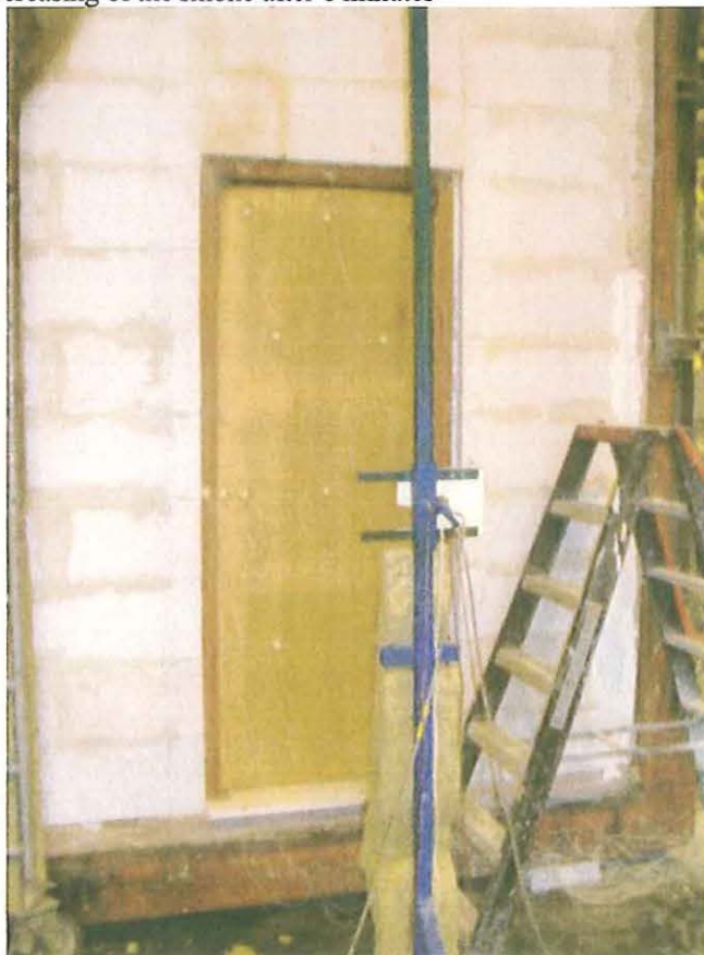
Photo 12: Door A covered with insulation and continued with door B
