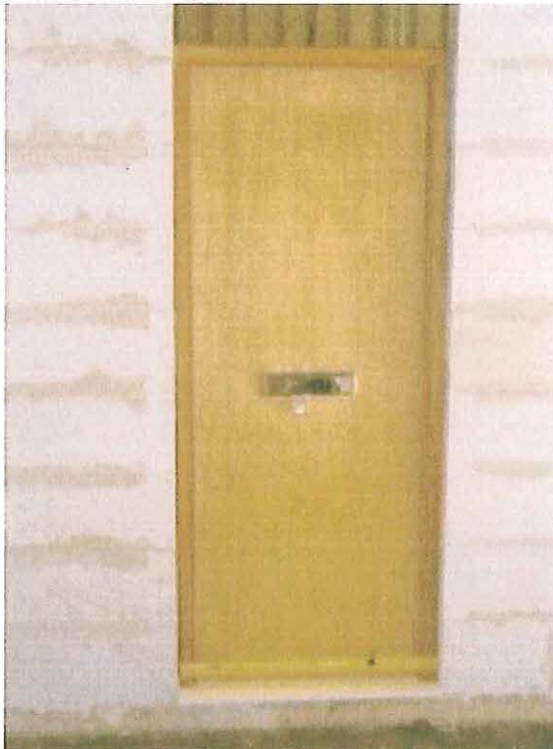
Photo 8: Door A with letterbox during assembly
