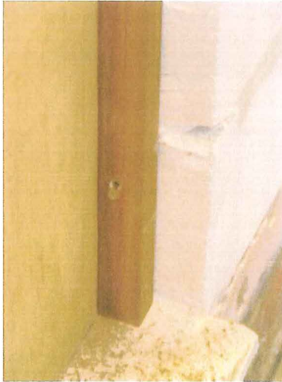
Photo 7: Fixing of wooden door frame
